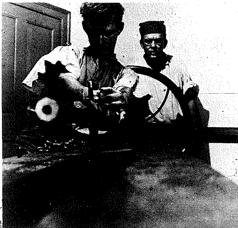
PLATE 178 Wallace Gusler and his assistant boring a barrel. (Photo courtesy of Colonial Williamsburg.)
