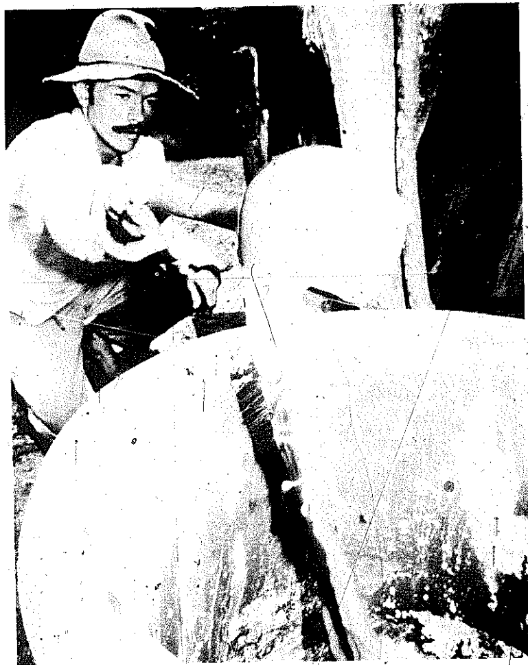
PLATES 208-209 The cave dirt was dumped on top of the straw in the V-vat, and water was poured over the dirt (Plate 208), picking up the soluble nitrates from the dirt and then flowing into the catchment trough. The "mother liquor" or "beer" was ladled into a container to be combined with the wood ashes (Plate 209). (Photos by Pete Lindsley.)
