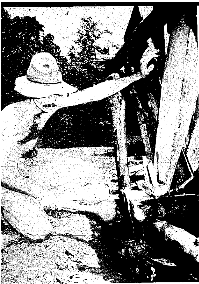
PLATES 208-209 The cave dirt was dumped on top of the straw in the V-vat, and water was poured over the dirt (Plate 208), picking up the soluble nitrates from the dirt and then flowing into the catchment trough. The "mother liquor" or "beer" was ladled into a container to be combined with the wood ashes (Plate 209). (Photos by Pete Lindsley.)
